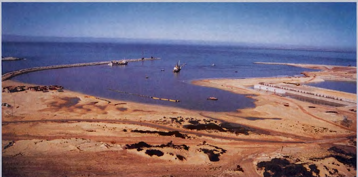
The Port of Ngqura Harbour under construction.
