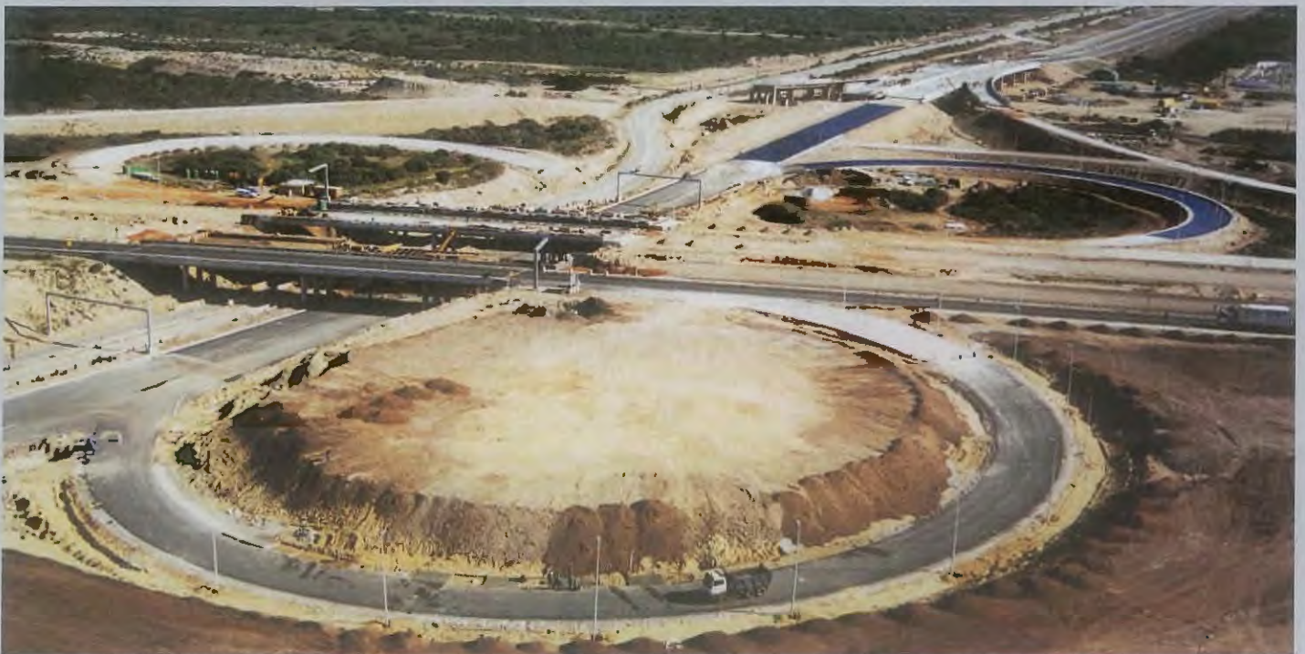
Aerial view of the N2 Doubling and the Neptune Road Systems Interchange.
