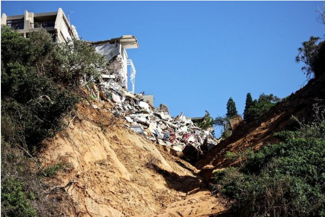
Side of apartment complex torn down by floods in Umdloti, Durban. Photo: RLS Southern Africa
