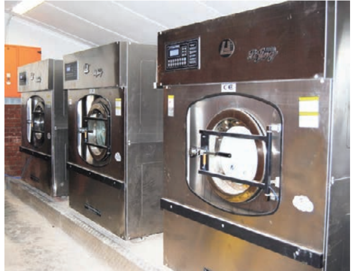
Mosa Engineering Services Recent Completed State Hospital Laundry Installation
