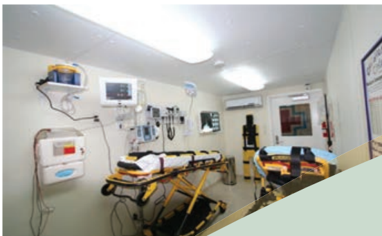
6m Container Interior (Trauma Response Unit)
