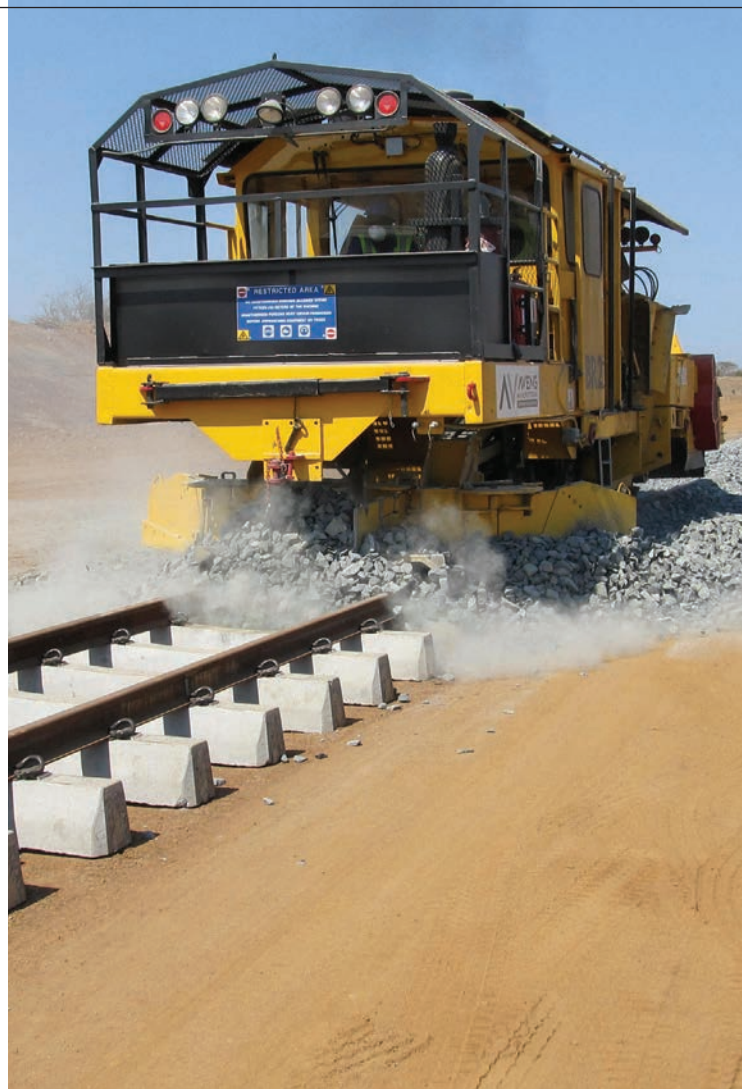
Moatize Coal Railway Line, Mozambique
