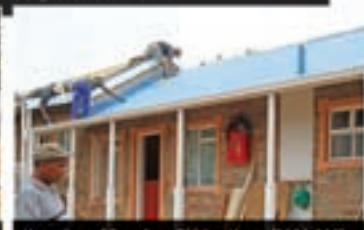
Upgrading of Swartberg Old Age Home (R338 000) in Dysselsdorp.
