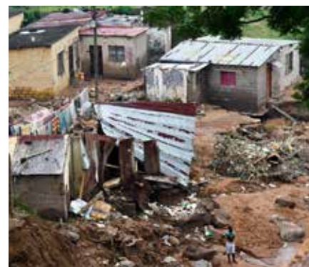
KZN flood damage
